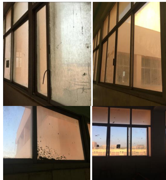
Picture 2: The current appearance of the building windows glass
