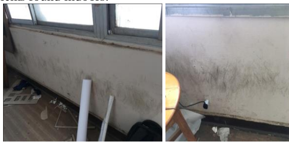
Picture 1: The current appearance of the building interior walls
