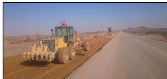
Figure (5) Earthwork operations from site.
