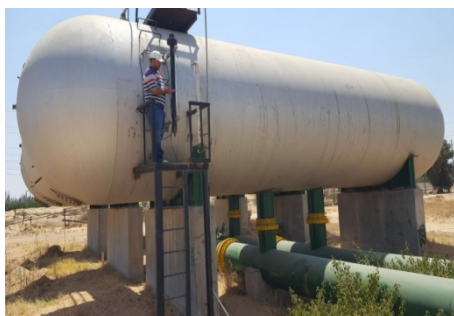
Figure 11. Air vessel.
